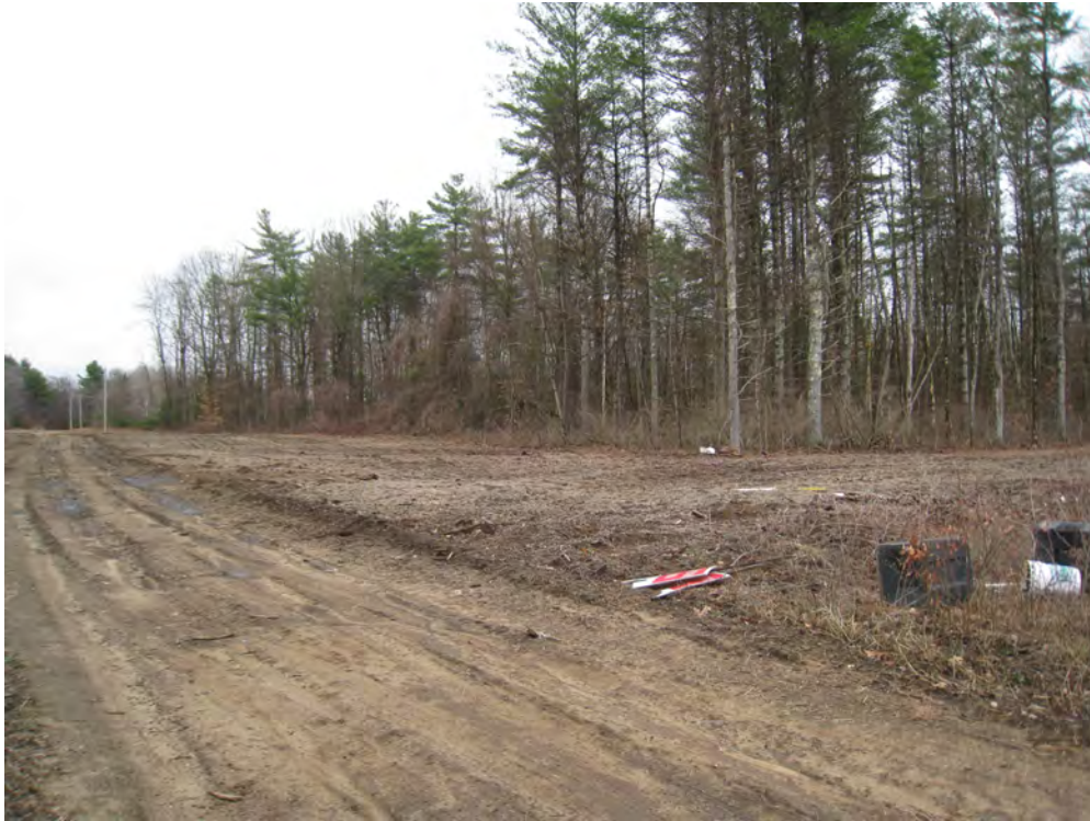
PHOTO 1: VIEW LOOKING SOUTHEAST AT PROPERTY FROM NORTHWEST CORNER
