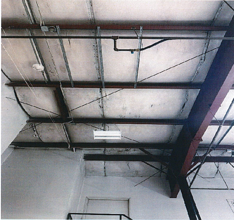
Bay ceiling above ambulance 5851
